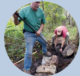
Stewards add rock steps to the Bog Brook Cove Preserve Ridge Trail, which will last much longer than wooden steps.
