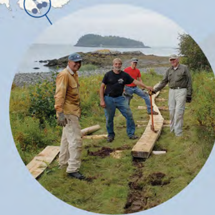
Volunteers replace old bog bridging at Western Head Preserve in Cutler.
